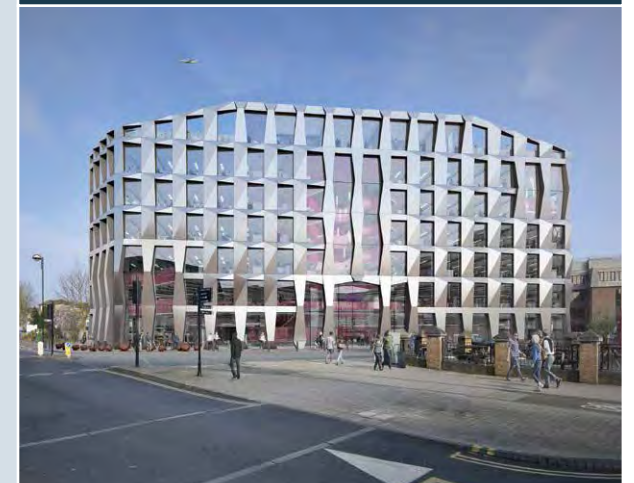
HOUNSLOW CIVIC CENTRE Being developed by Bouygues Development
